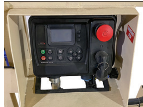
Weatherproof Ignition Panel
